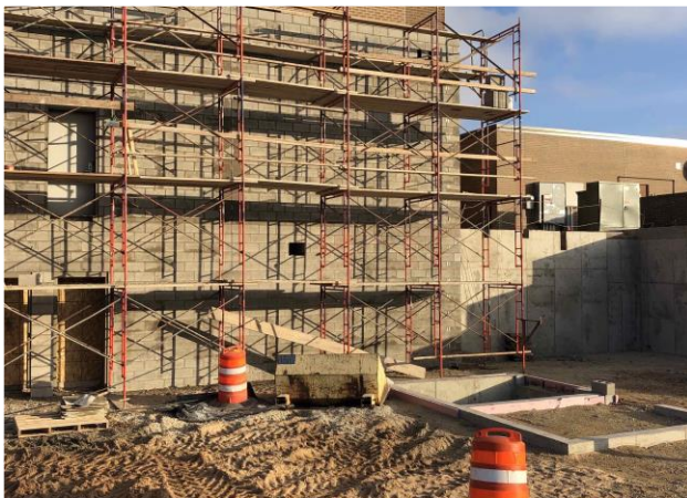
Erecting masonry fire wall at Addition A
