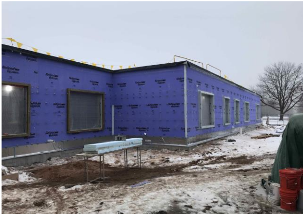
Installed blocking & flashing at Addition C
