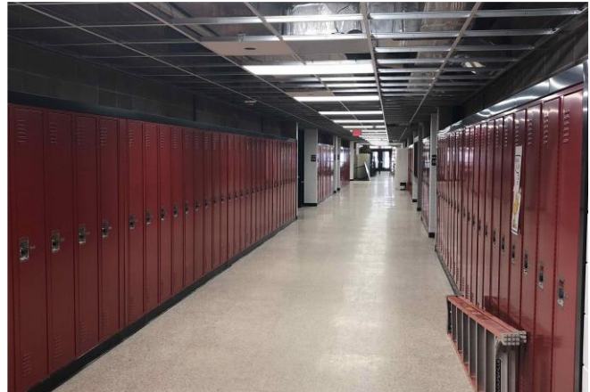
Installed Corridor ceiling grid and lighting
