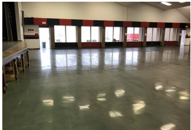
Polished concrete completed in Commons
